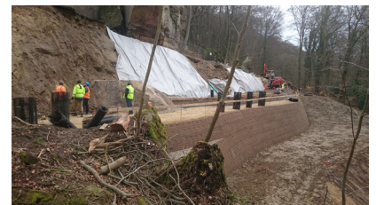
Figure 12: Rock outcrop integrated into the stabilisation system.
